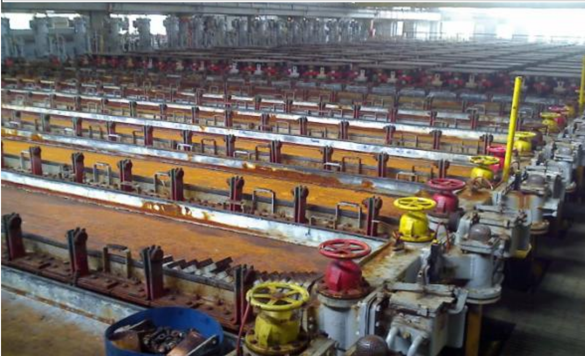
First stage of operations
