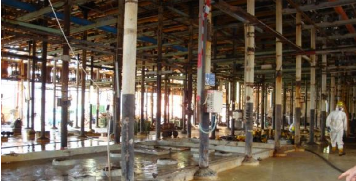
Floor of cell room regularly washed down
