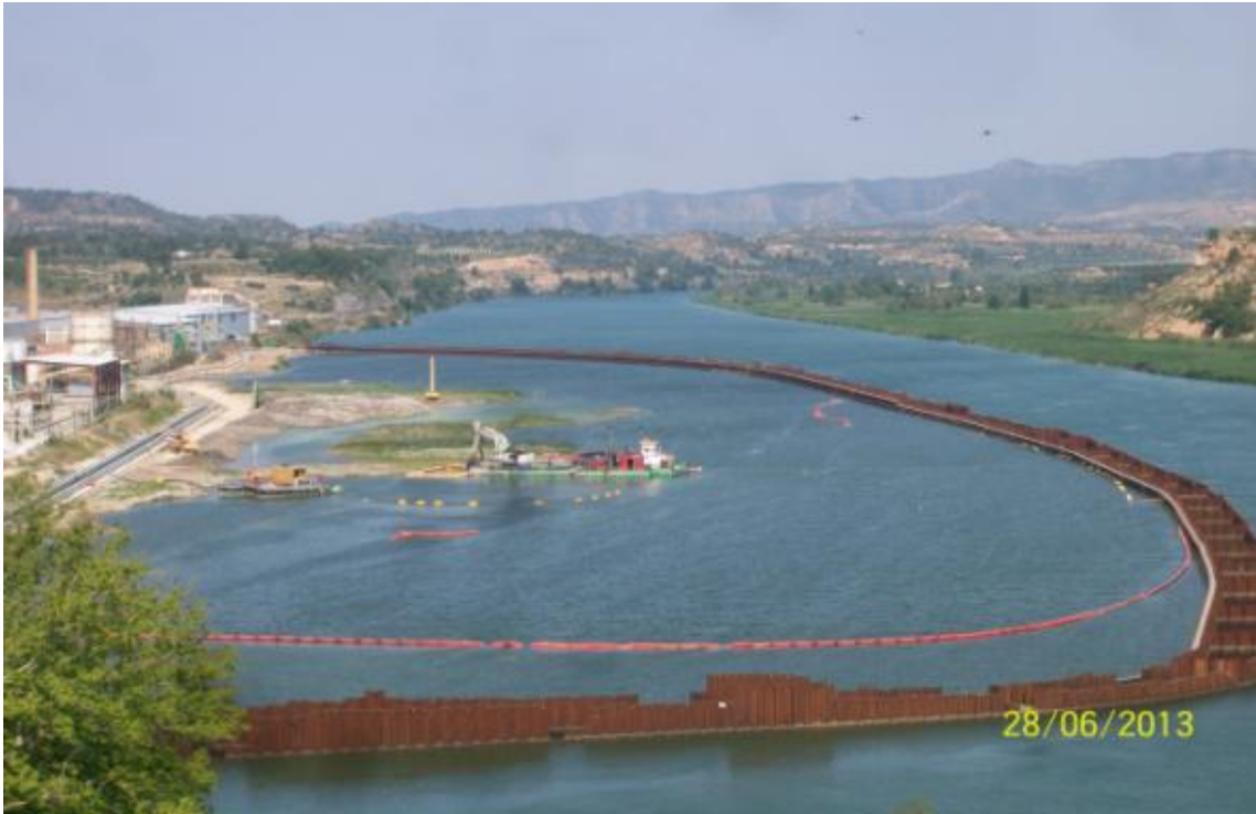
Dredging activities inside the sheet piling
